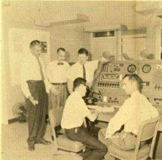
FAA PERSONNEL —Personnel of the Federal Aviation Administration are shown looking over new equipment installed in the second floor of Pierre's new airport terminal building. Left to right (standing) are M.A. Simons, Station Chief at Pierre, L.S. Rusk, of the FAA Kansas City office, and George Kniska, Chief Air Traffic Manager for the FAA from Kansas City. Seated are Don Pater and Don Angle, both of the Pierre FAA office.
